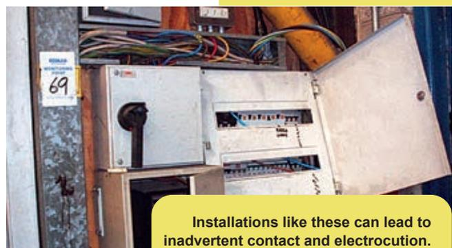
**Installations like these can lead to inadvertent contact and electrocution.**
