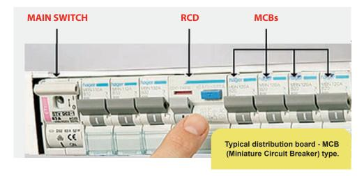
Check that your RCD is working correctly by pressing the test button marked 'T' or 'Test'. Remember this will cut the power to all socket outlets so make sure no essential work is being done at the time.
