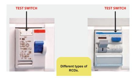
If it is working, power to the socket outlets will immediately switch off. If the RCD fails to trip, it should be replaced immediately by a registered electrical contractor.
