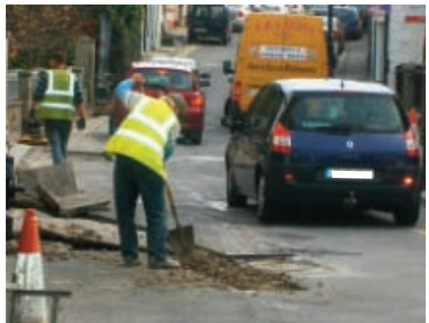
*Example 4 A worker carries out work activity with his back to oncoming traffic on the roadway. No arrangements are in place to control the movement of public vehicles close to site workers.*
