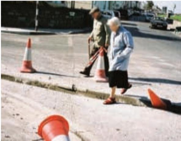
*Example 1 Inadequate protection of this construction work on the roadway, resulting in elderly road users having to step over an open trench. Adequate signing, lighting and guarding measures should have been implemented to prevent this situation occurring.*
