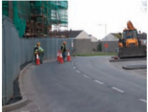
*Example 2 Three workers carrying out construction work at busy bend on roadway. Insufficient and inadequate signing, lighting and guarding measures in place to protect the work crew and other road users.*
