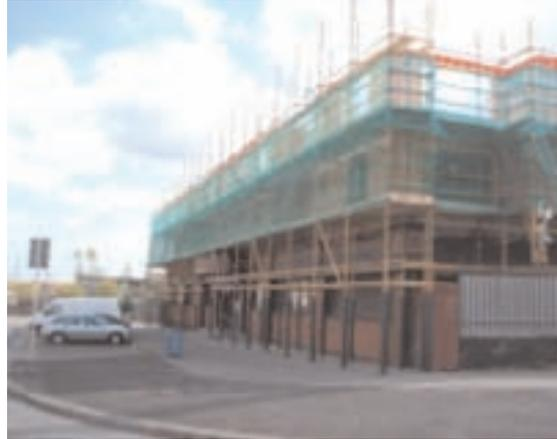
*Photograph 11* Scaffold erected on a wide footway.
