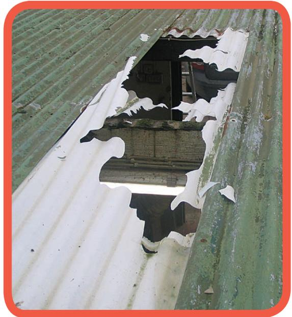
Ensure all the work areas and access platforms are fitted with guard rails. If this is not possible, install safety nets or air bags underneath the roof or use a harness system. Where harnesses are used, make sure you are trained in their use. It's important that they are stored and maintained properly, that they have adequate anchorage points and they are properly used – through appropriate discipline, training and supervision.
