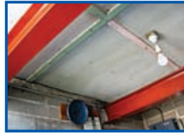
AIB ceiling panels in lift motor room
