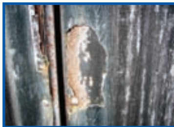
Galbestos - asbestos bitumen layer to metal corrugated sheeting
