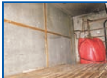
Asbestos cement wall panels in hot press
