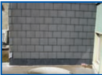
Asbestos cement flat profile roof tiles
