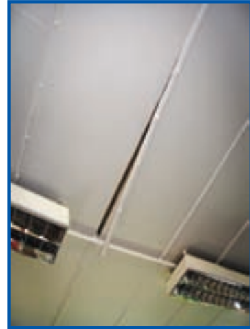
Asbestos cement ceiling panels
