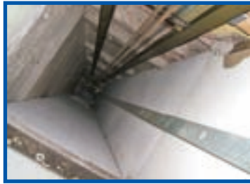
AIB lining to dumb waiter shaft
