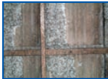
Asbestos spray coating to underside of asbestos cement corrugated roof
