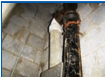
Asbestos cement flue pipe
