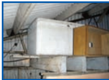
Asbestos cement water tank in attic
