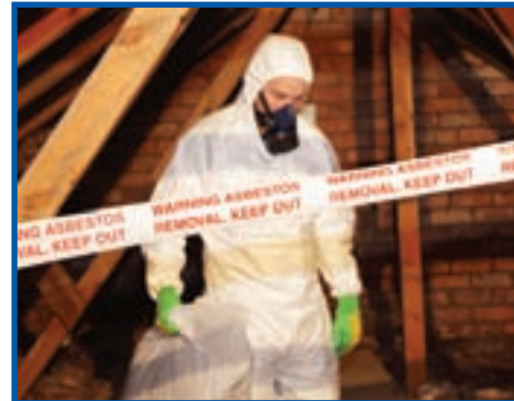
Asbestos worker using orinasal respirator (half mask)
